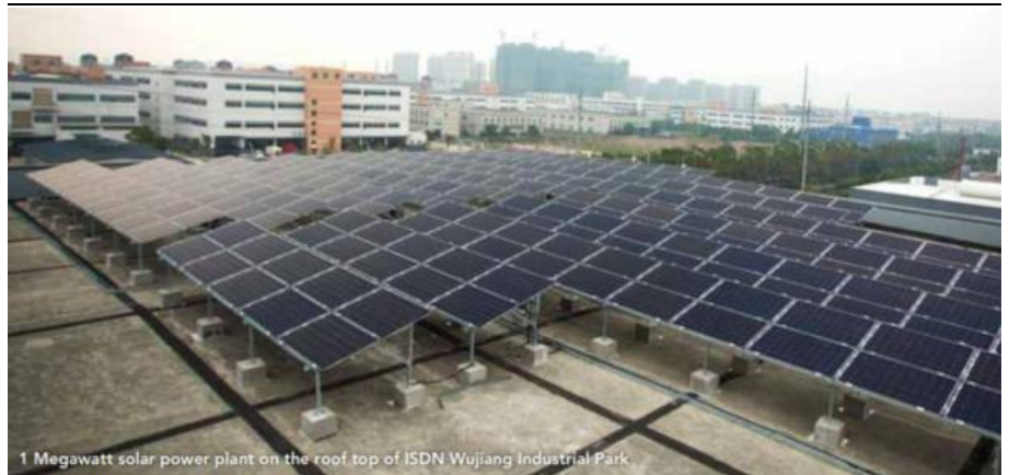
Figure 4: ISDN's 1 MW solar power plant in Wujiang Industrial Park
