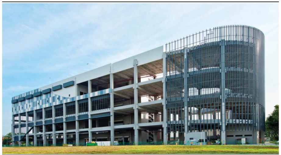
Figure 5: 3 Tuas Avenue 2, Singapore
