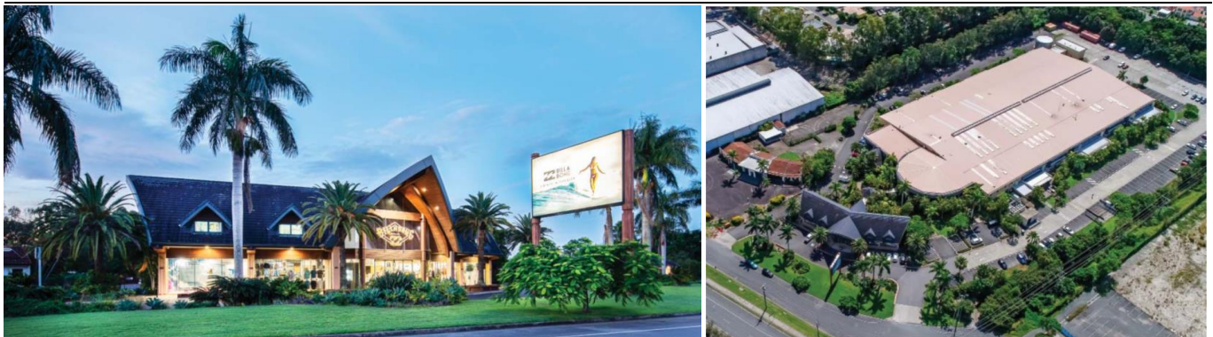
Figure 2: Boardriders Asia Pacific HQ, 209-217 Burleigh Connection Road, Burleigh Waters, Queensland, Australia
