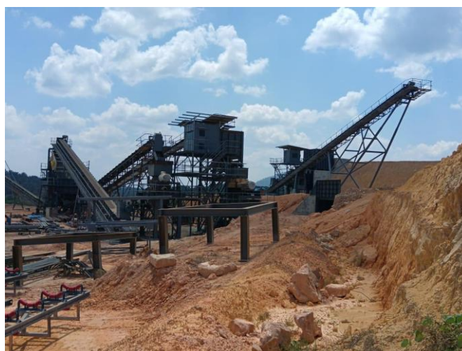
Figure 6: Seri Bandi processing plant under construction
