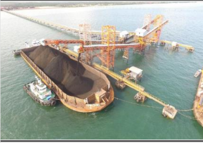
Figure 10: Direct barge loading at BIB
